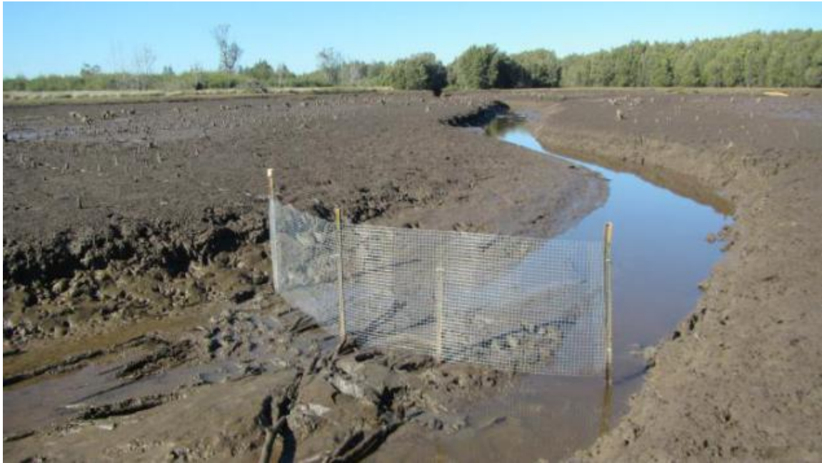
Image 10. A repaired MPED ready to do its job.
