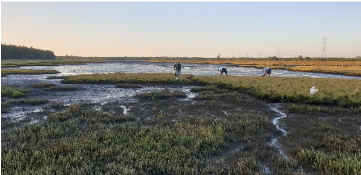
Figure 8. The work at Milham Pond starts at the highest end of the system. The finish line is far away in the distance.
