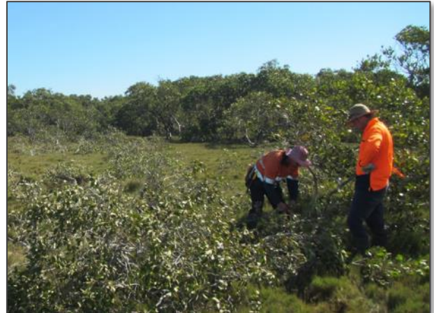
Contractors moving quickly across the work area. A more open saltmarsh will better suit night-time roosting of shorebirds
