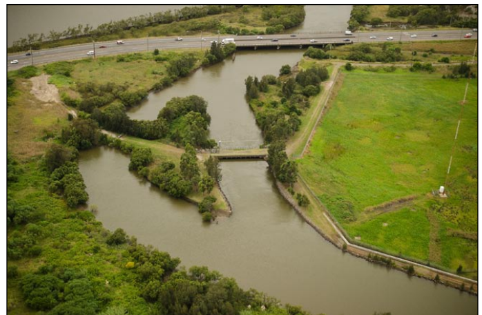
Extent of saline water increasing in Hexham swamp (top) and view of Ironbark Creek, tributary of the Hunter River (below) - photos by CMA
