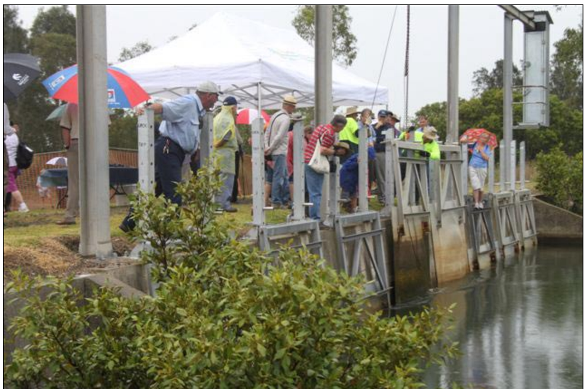
Opening the tidal gates on Ironbark Creek in December 2009. Photo: Ann Lindsey
