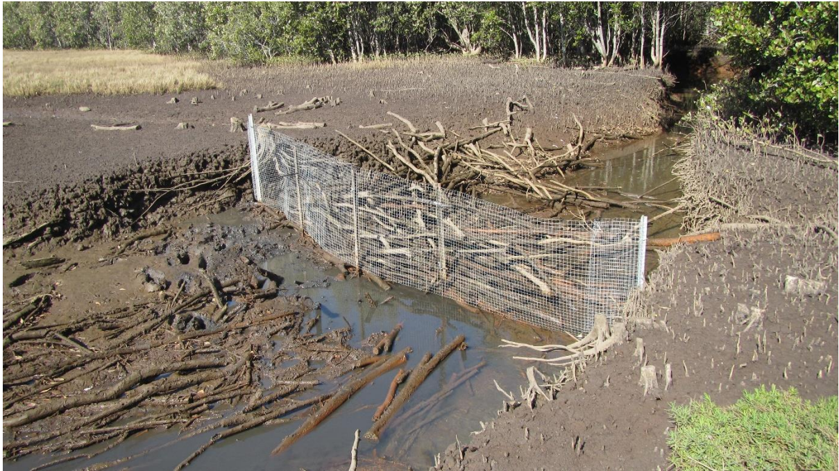
Figure 14. New mesh installed and ready to trap the next wave of mangrove seeds.
