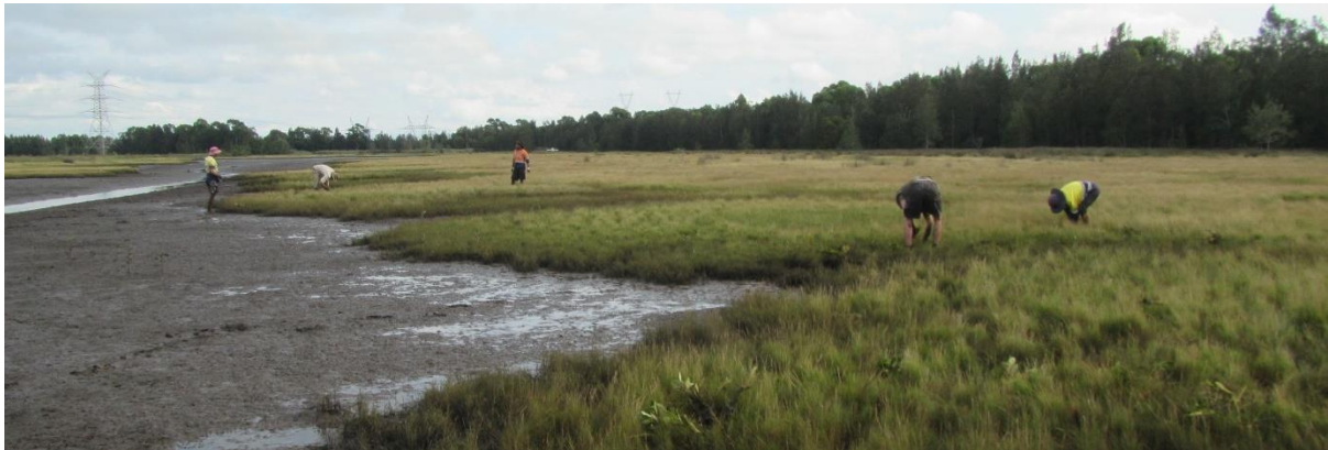
Figure 7. Combination of volunteers and contractors hard at it near Neville's Nook.
